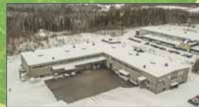
GTP Tikomet - Jyväskylä, Finland Zinc Recycling
